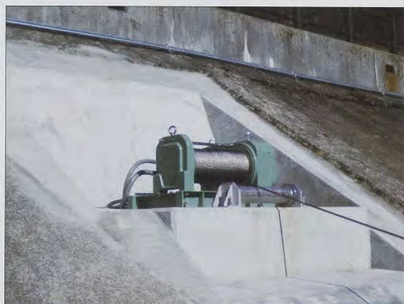
Mooring facility of Dam Lake
