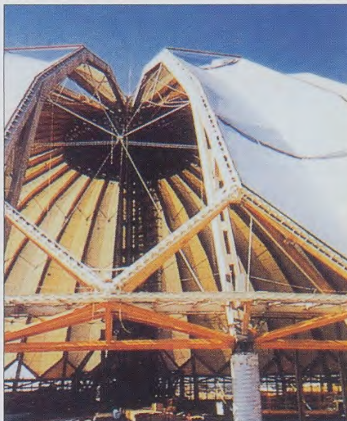
For hoisting equipment and nets in the dome
